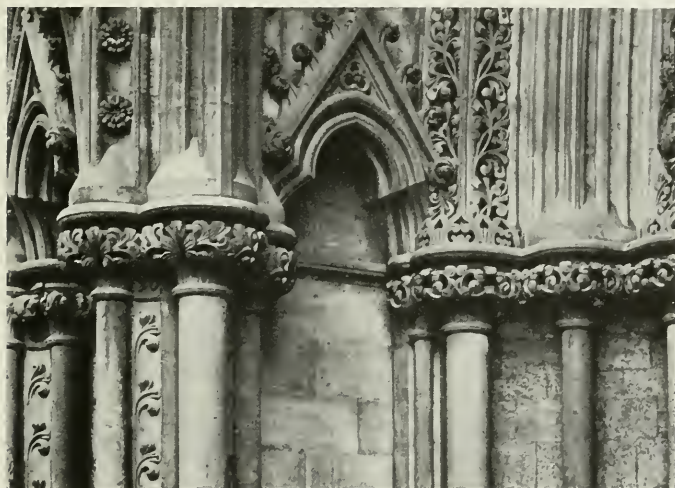
39. Modern Carving from Restoration of Porch to North Transept, Westminster Abbey.
